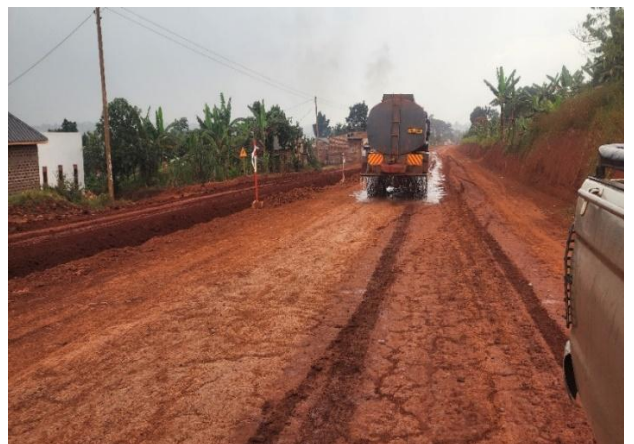
Dust suppression; section of Bukasa-Sentema-Kakiri Road
