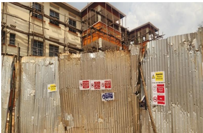
Fenced construction site at Buloba - Kitawuluzi Health Centra III.
