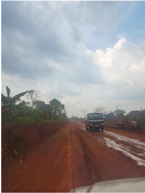
Upgrade of Bukasa-Sentema-Kakiri to Bituminous Standards
